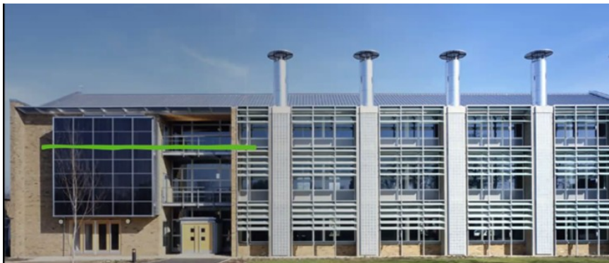
Solar (thermal draught) and photovoltaic chimneys
